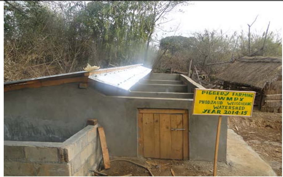
Piggery Shed in West Khasi Hills District
