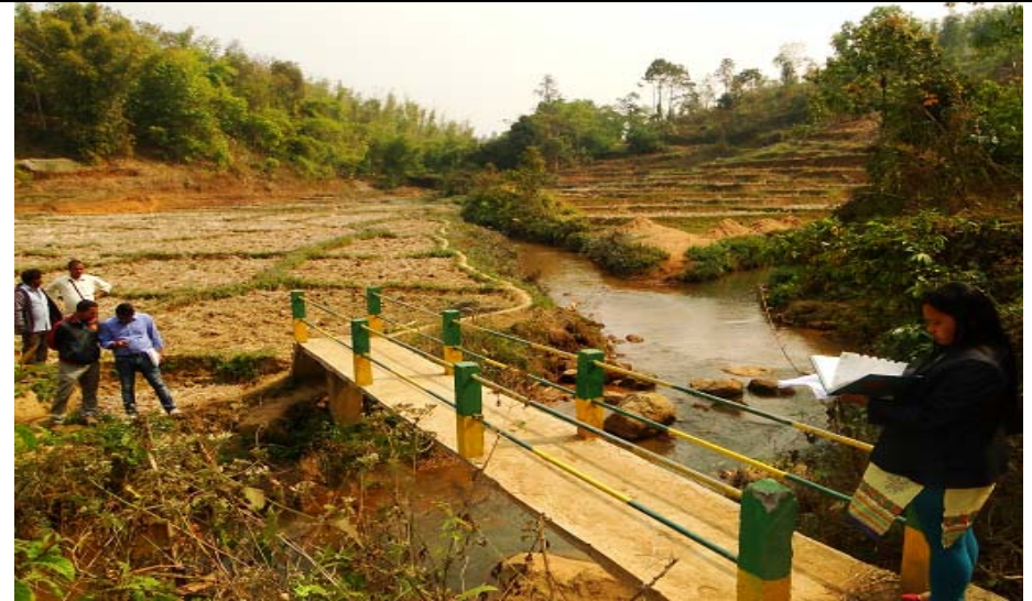
R. C. C. Foot Bridge in Ri-Bhoi District
